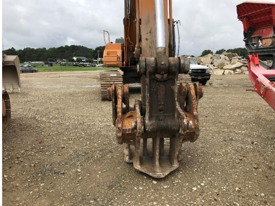
Figure 12.12.13 The Breaker for Initial Breakdown the Slabs and Remove Rebar
