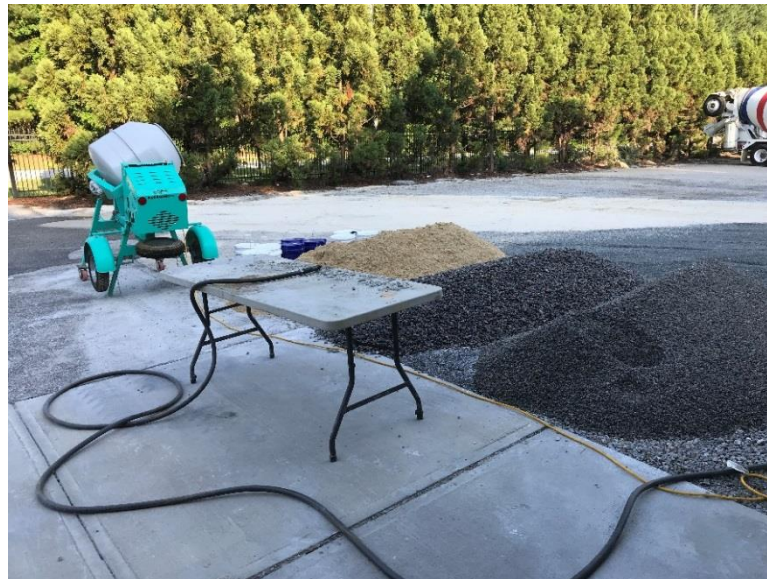
Figure 5.1.1 Equipment and Materials are Ready for Concrete Batching
