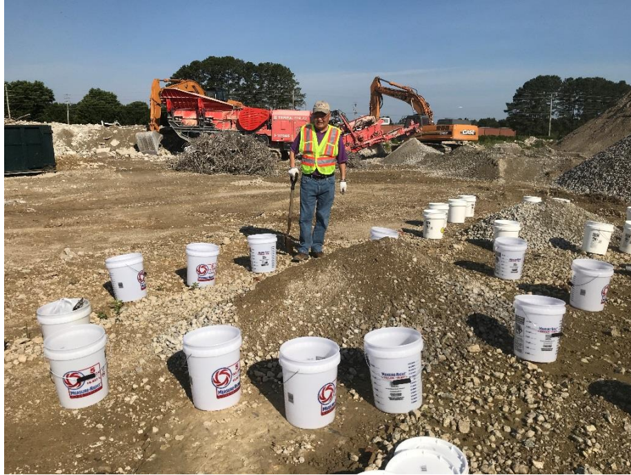
Figure 12.12.19 RCA Sampling (Division 2) at S.T. Wooten's Wilson Plant
