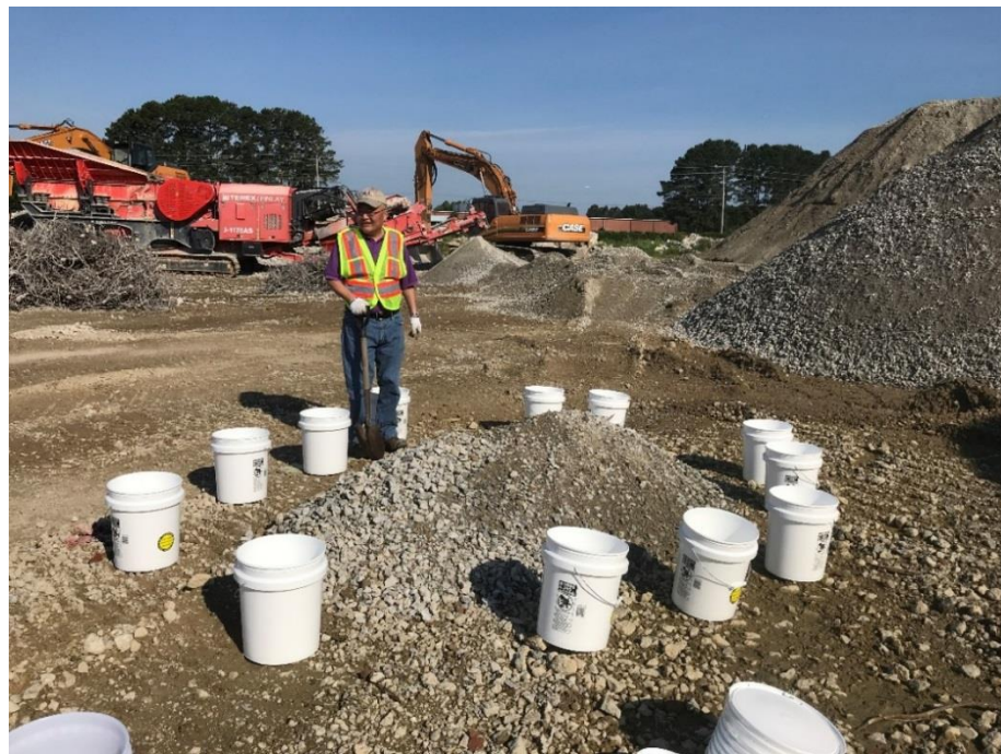
Figure 12.12.20 RCA Sampling (Division 3) at S.T. Wooten's Wilson Plant
