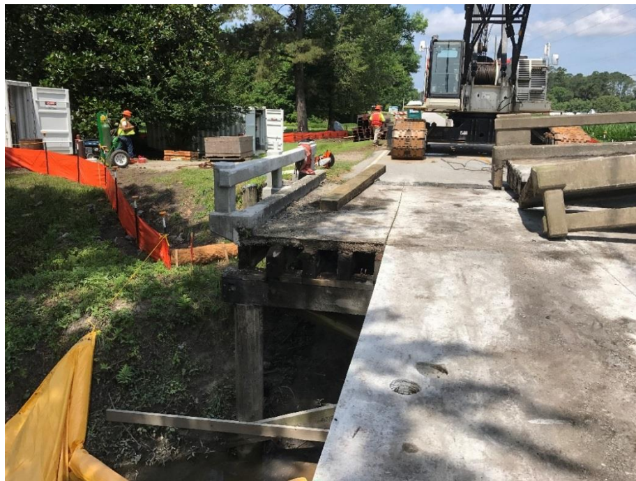
Figure 12.12.4 Bridge Removal Construction Site in Division 2
