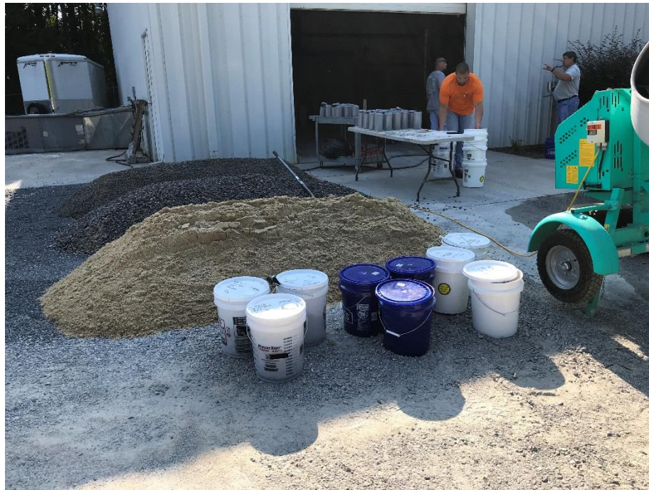
Figure 12.12.42 Materials and Equipment Were Ready
