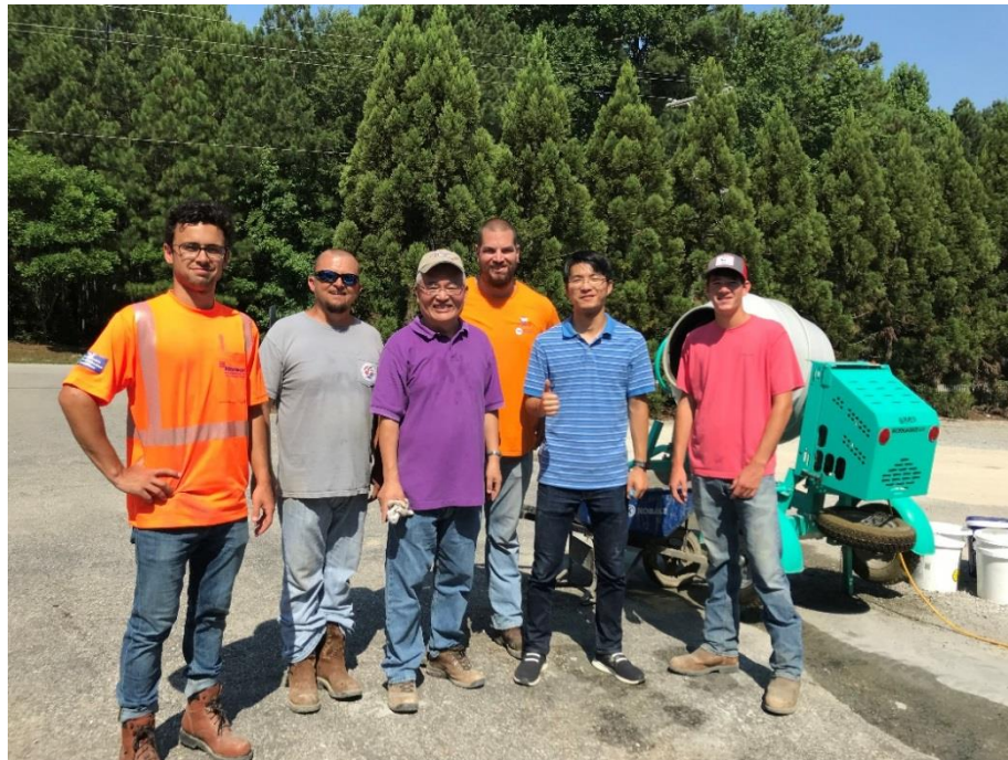
Figure 12.12.36 The Concreting Team Was Ready for Concrete Batching
