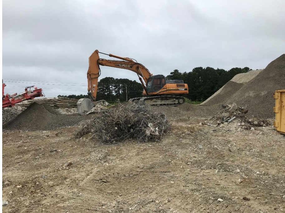
Figure 12.12.15 Reinforcing Steel is Removed
