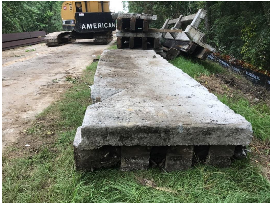
Figure 12.12.6 Slab to be Transported to Crushing Plant in Wilson, NC (Division 3)
