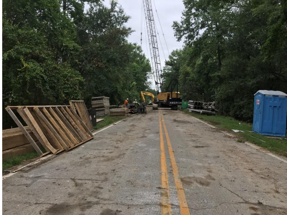
Figure 12.12.5 Bridge Replacement Site in Division 3
