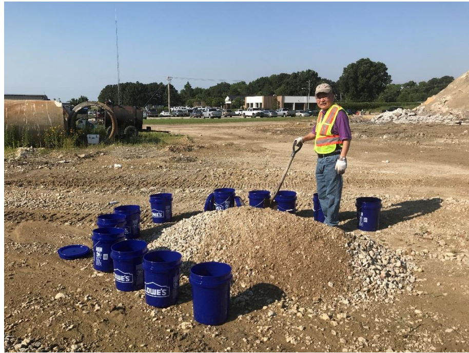
Figure 12.12.18 RCA Sampling (Division 1) at S.T. Wooten's Wilson Plant
