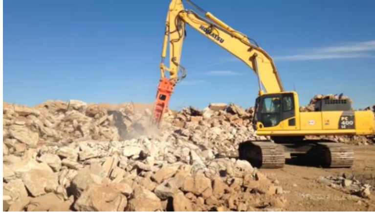
Figure 4.2.1 Pulverizer Used to Size and Remove Rebar
