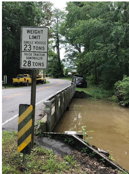
Figure 12.12.2 Bridge in Division 1 Where the Concrete Slab Was Saw Cut
